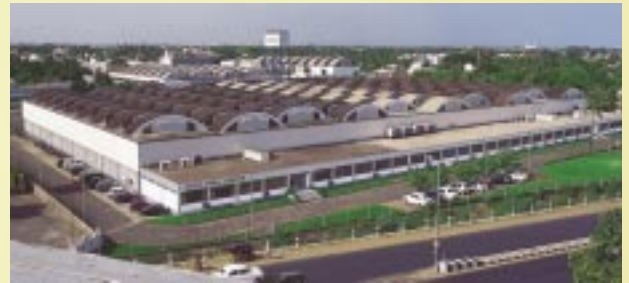
Administrative Office and Manufacturing Plant at Manapakkam
